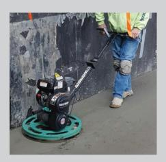
Allows finishing within 7/16" of any obstruction
